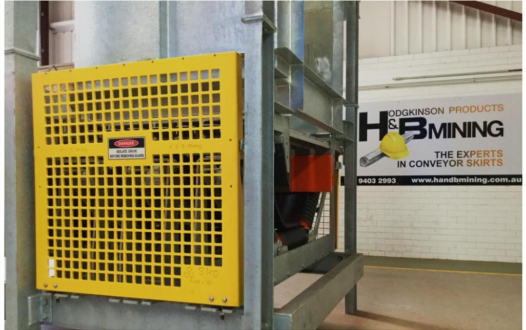
High density polyethylene (HDPE) conveyor guarding offers a lightweight, corrosion-free, low maintenance alternative to conventional guarding.
