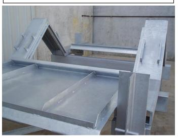
DUST COVERS FULLY OPENED AND RESTING ON DUST COVER SUPPORTS. FLAT COVERS ACT AS A W/WAY AND PLATFORM TO AID WITH ACCESS FOR INSPECTION AND MAINTENANCE
